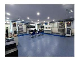
• The trainee will be able to study various features of panel operation. The trainees will be exposed to troubleshooting the failures created. The trainee will be able to study different types of relays and their purpose.
